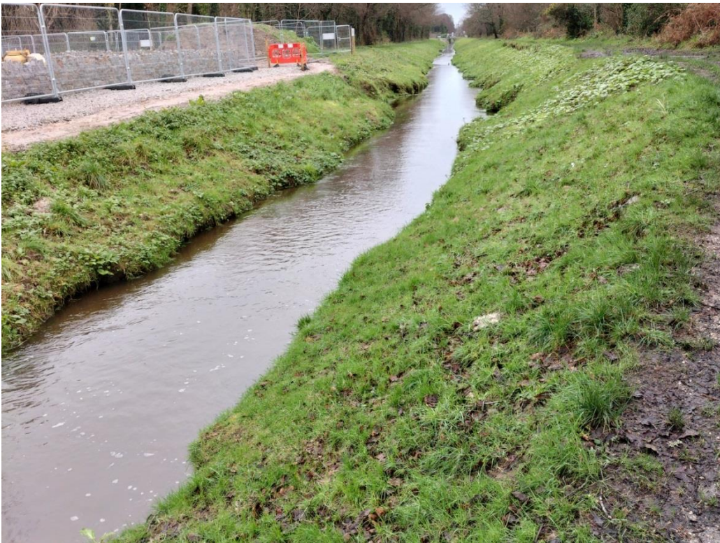
Par Canal at Middleway showing StARR project engineering works on left.
